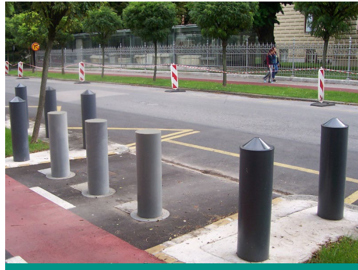
Combination of fixed and automatic bollards.
