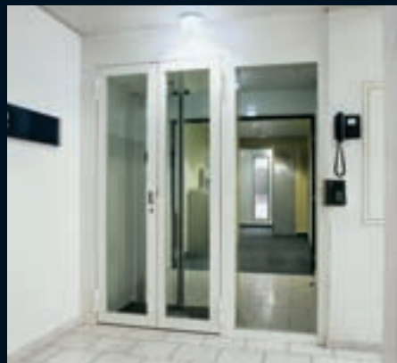
Interlocking doors type RENO with R30-requirement as a staff entrance from a staircase-hall.
