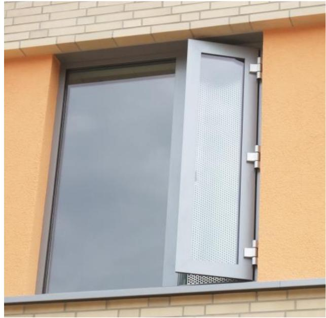
Window combination: fixed window field at the left side in combination with a side hung outward opening window leaf, inside a perforated sheet.
