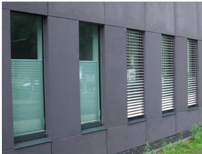
On the left side: 2 blinds are installed inside the glass, next to them on the right side the blinds are installed outside in front of the windows.
