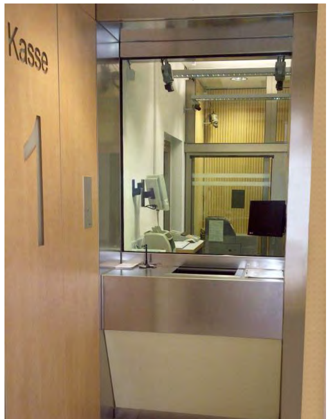
External speaker integrated in the ceiling and microphone integrated in the frame, aluminum cover is sandblasted.
