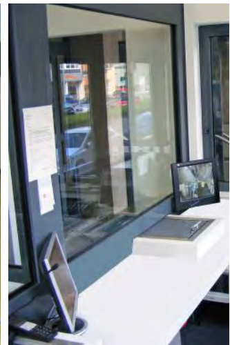
Guard room in the entrance hall of a courthouse. Equipped with transaction window incl. exchange drawer, intercom, door control system, video surveillance.
