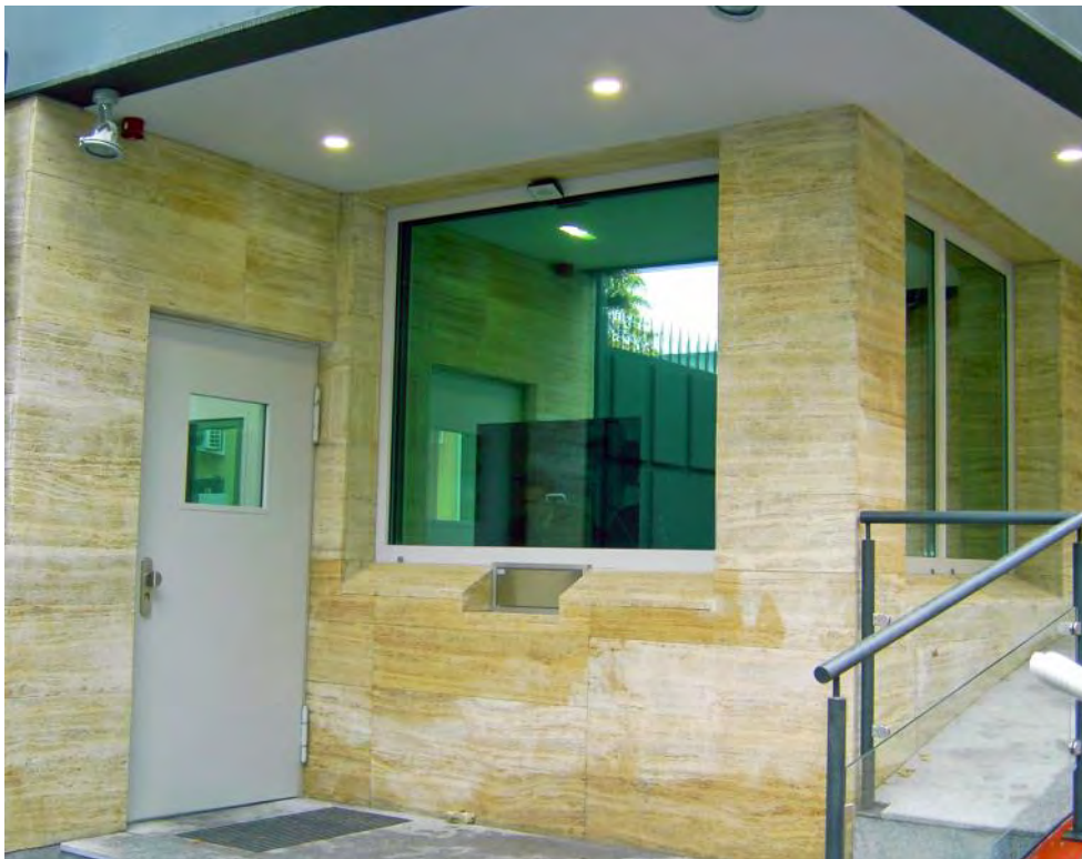
Entrance area of a German embassy, transaction window with flush-mounted exchange drawer, glazed security door.
