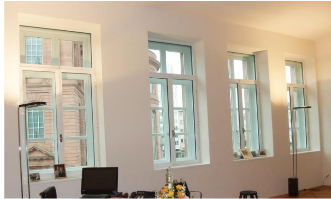
Secondary window for the interior: window with tilt and turn wing .
