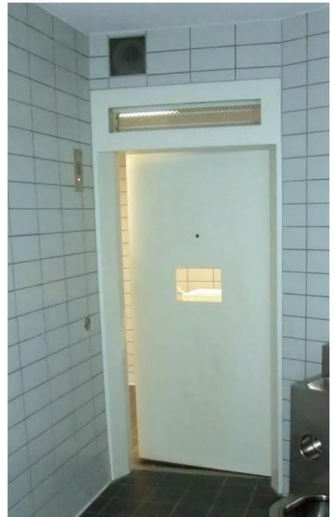
View inside the cell: SÄLZER S4-Z door with fanlight. The door is mounted flush to the wall inside the cell. Therefore no protruding edges and no basis for any injury or suicide attempts.
