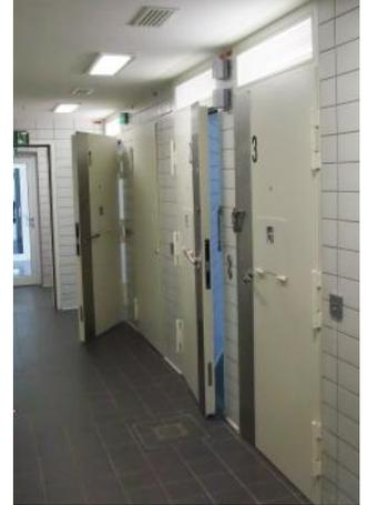
Cell section of a police station. Detention doors with stainless steel covering, food passers, security chains and quick release fasteners.
