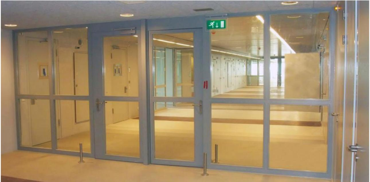
The door is generously glazed despite forced entry resistance in RC4 and anti-panic hardware according to DIN EN 179.
